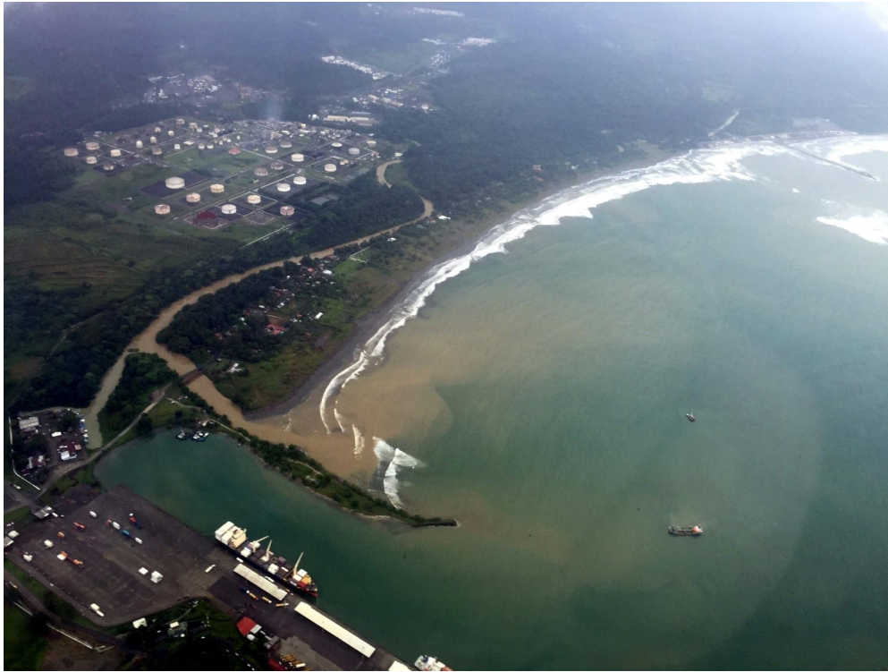
Figure 7. Overview of the project zone during a day in August . Source: BICA Consults
