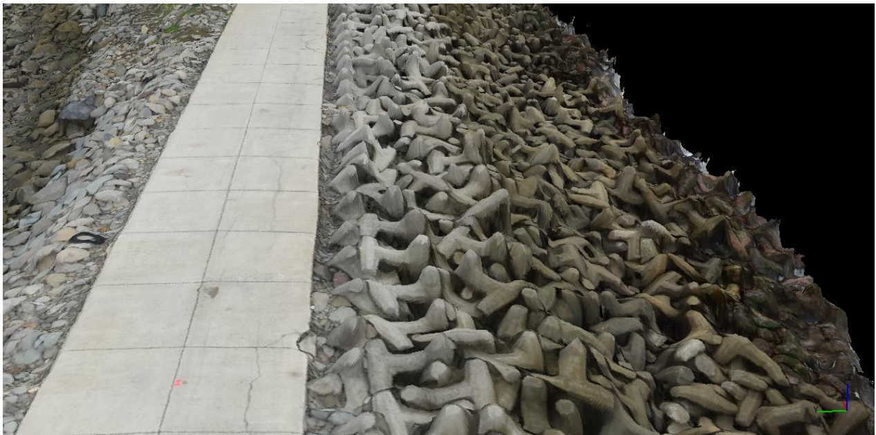
Figure 5. 3D reconstruction of the Caldera breakwater, Costa Rica
