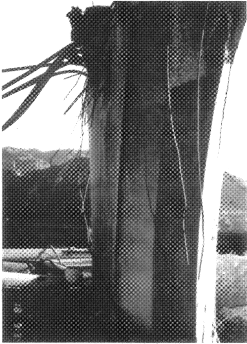
Fig. 5.6: Bent 3 of Interstate 5/Route 14, South Overhead
