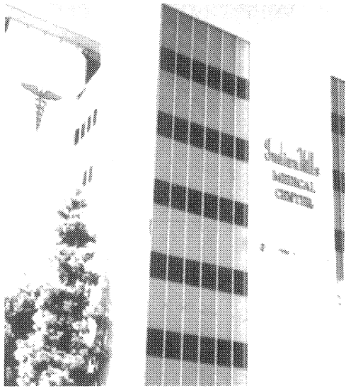
Fig. 6.17 Shear Wall Damage at Indian Hills Hospital
