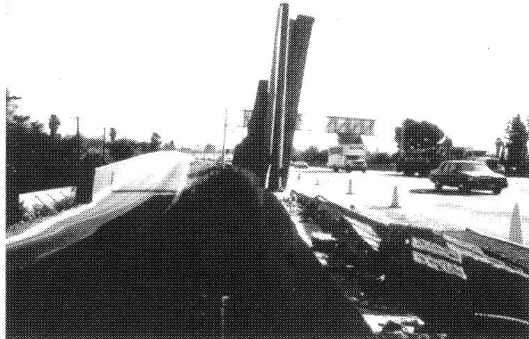
Fig. 5.25: Sound Walls at Route 101 near Interstate 405
