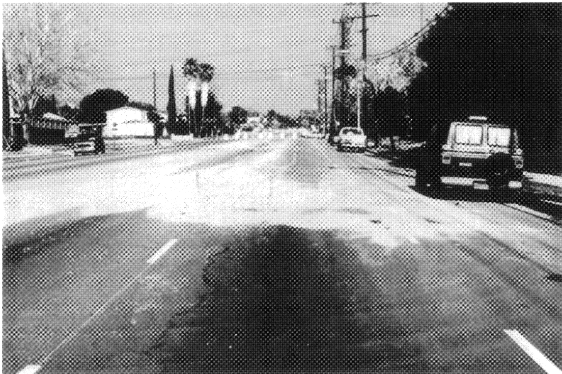
Fig. 4.10: Evidence of liquefaction and lateral spreading, northeast Northridge
