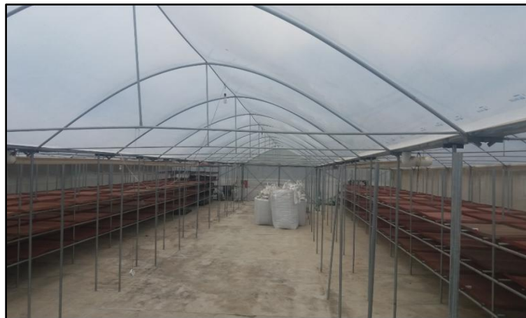
Fig 2. Distribution of trays for drying coffee inside the solar dryer
