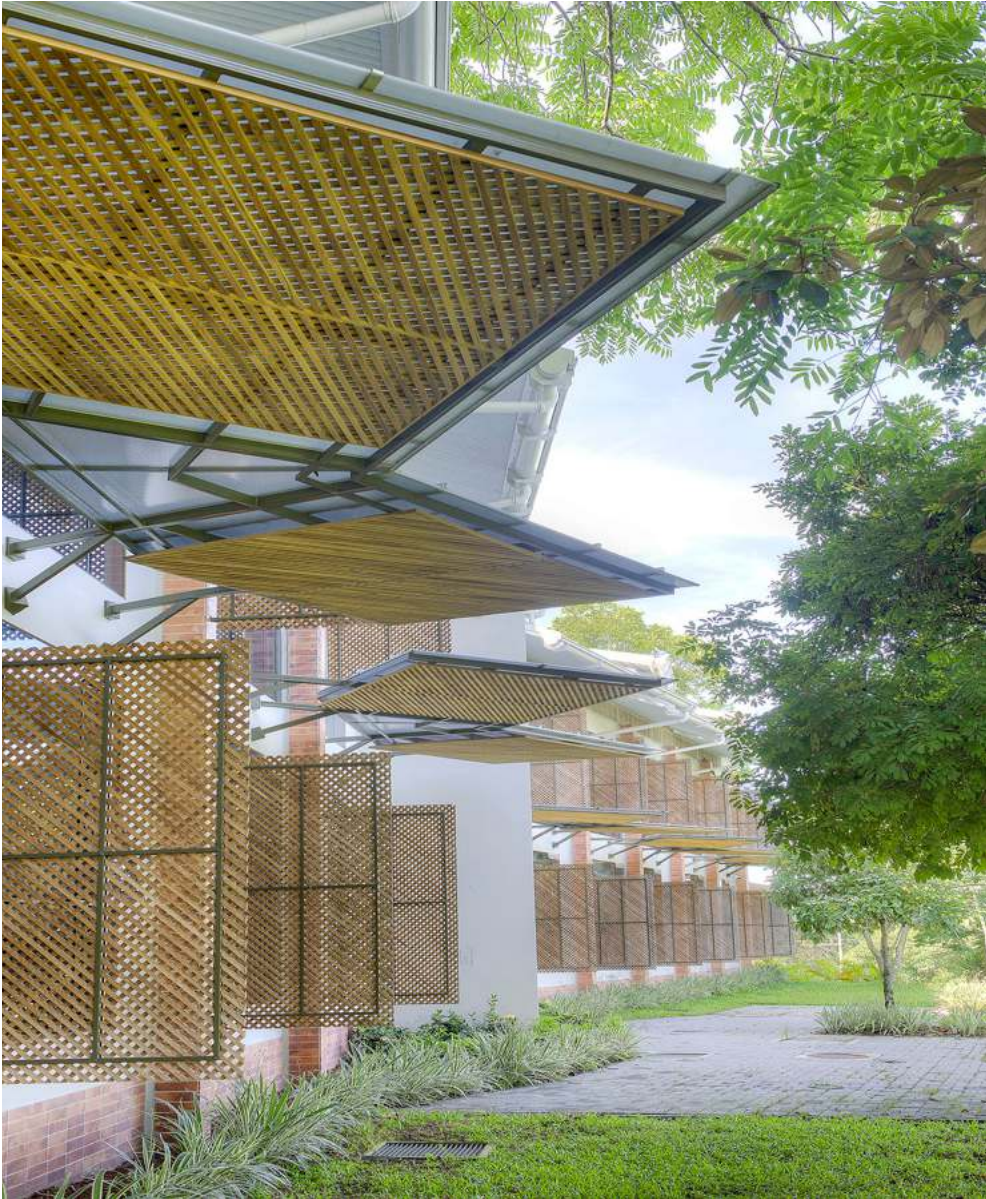
Figure 7: Instituto Centroamericano de Administración de Empresas Building, by Bruno Stagno, La Garita, Alajuela, Costa Rica, 2015.
